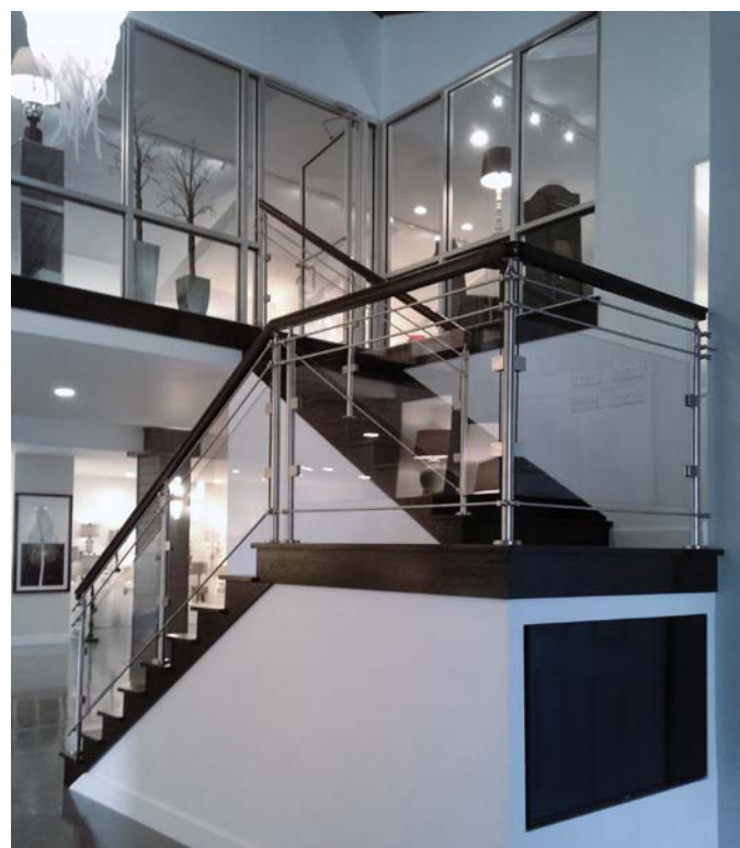
Stainless Steel Glass System with 1/2" Round Bar
